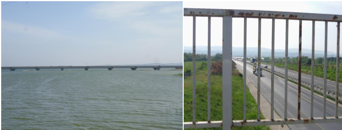
Figure 6: O-3 (E80) road cuts through the lake
